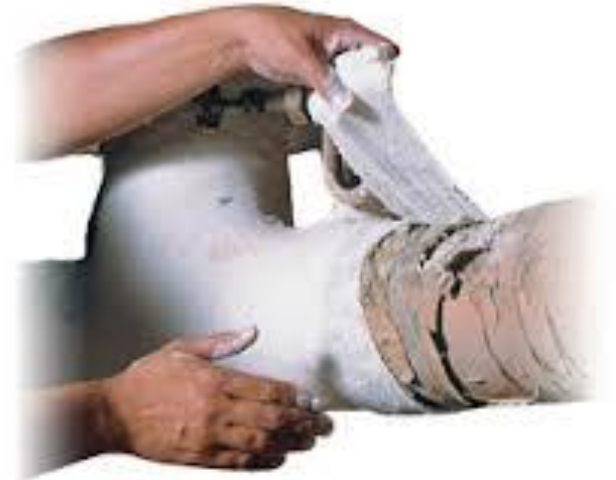
Boilers and Thermal Insulation
